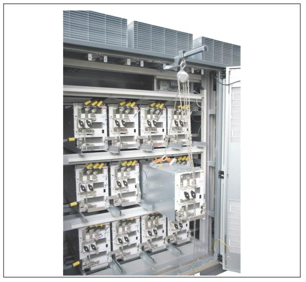
11. Lift again the blocking bar of the front lock, pull the power module completely out of the support module beam and lower it.
